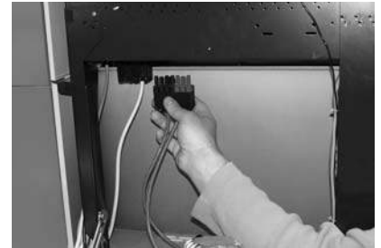
Fig. 128 Disconnecting the blower plug
