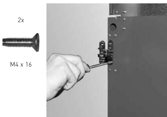
Fig. 59 Fitting both hinges on cladding door
