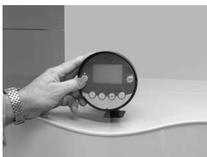
Fig. 137 Switching off BioWIN
