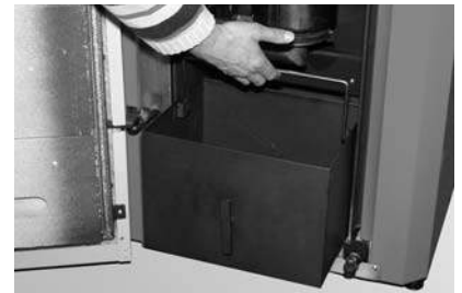
Fig. 110 Removing ash pan
