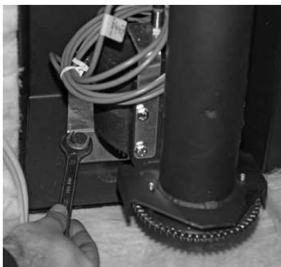
Fig. 16 Unscrewing transport attachments from boiler
