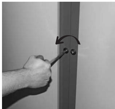
Fig. 75 Closing the cladding door with the key
