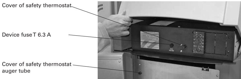
Fig. 145 BioWIN control panel cladding raised, combustion chamber door open
